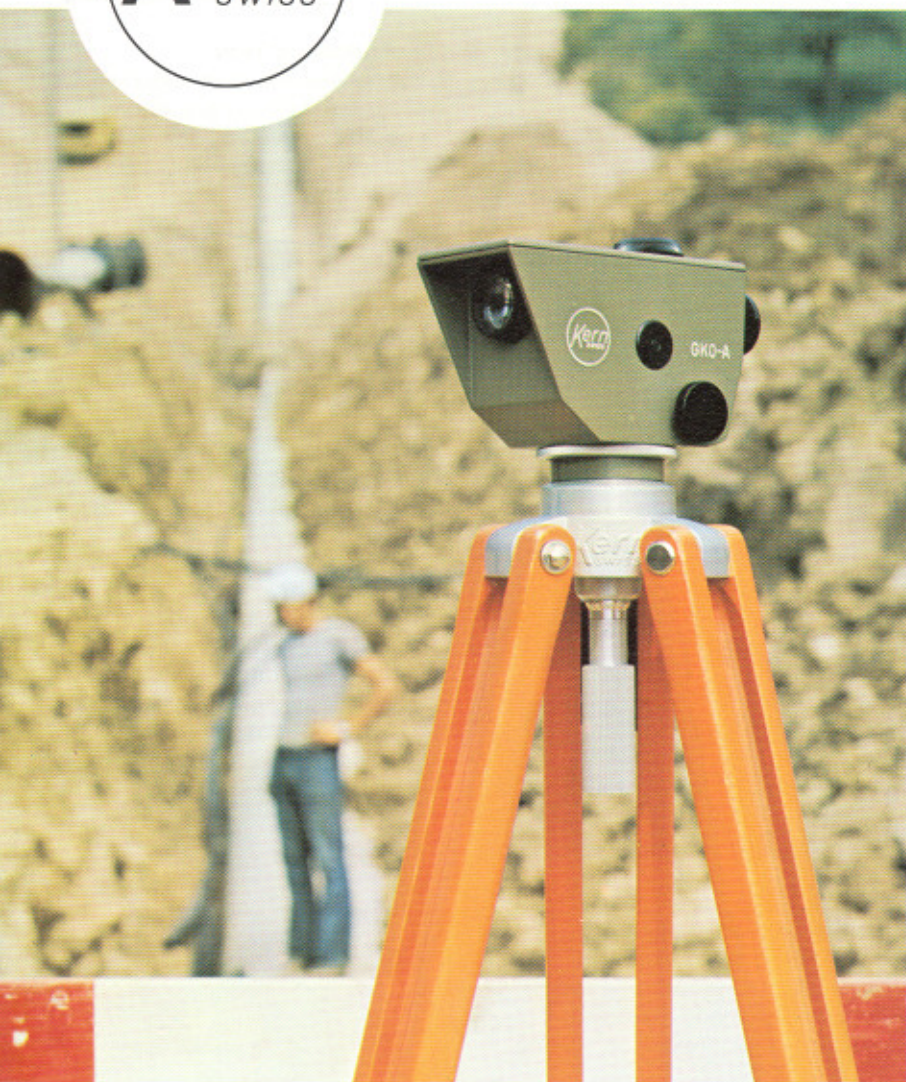
Checking measurements at the natural gas pipeline Netherlands-Italy
