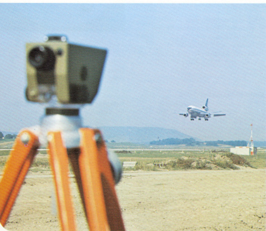
Leveling on a runway under construction at the Zurich Intercontinental Airport
